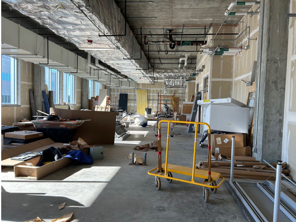
Fig. 2: Southeast Portion of Third Floor to Be Completed in FY2026
