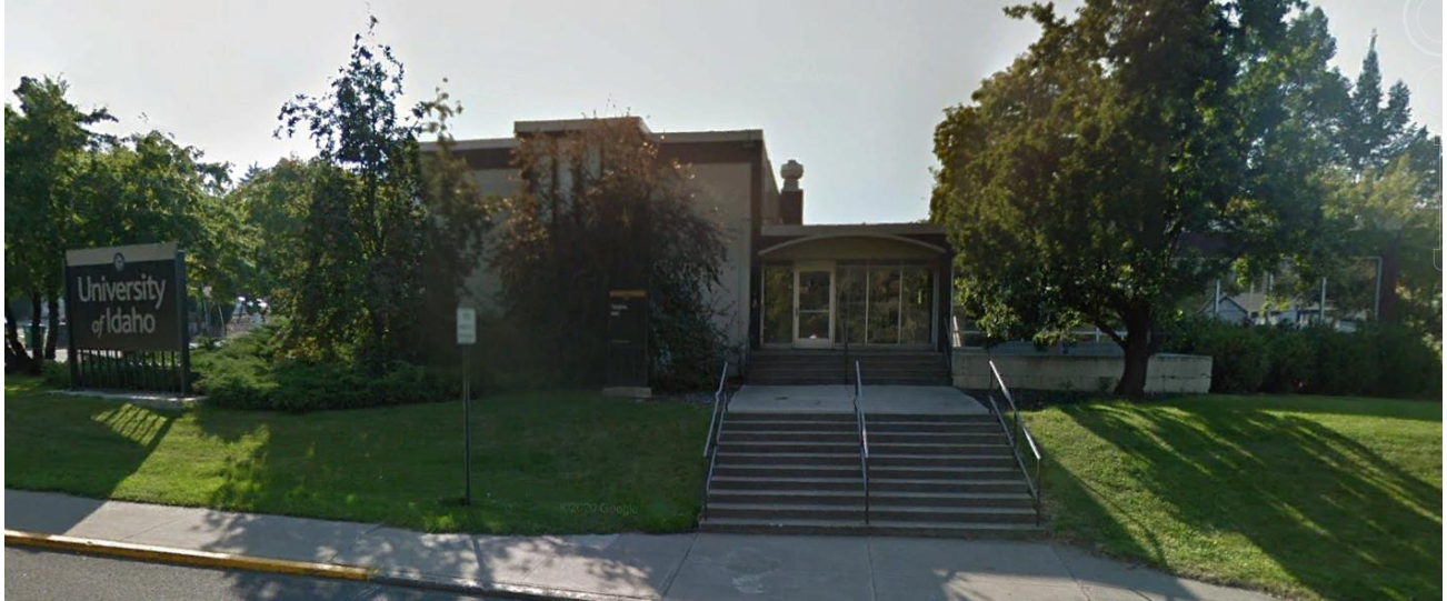
Existing Condition, Targhee Hall
