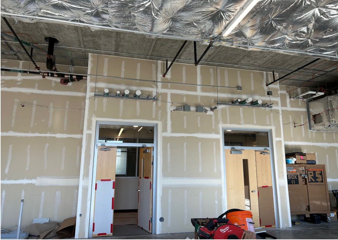
Fig. 4: Additional Unfinished View of Third Floor to Be Completed in FY2026
