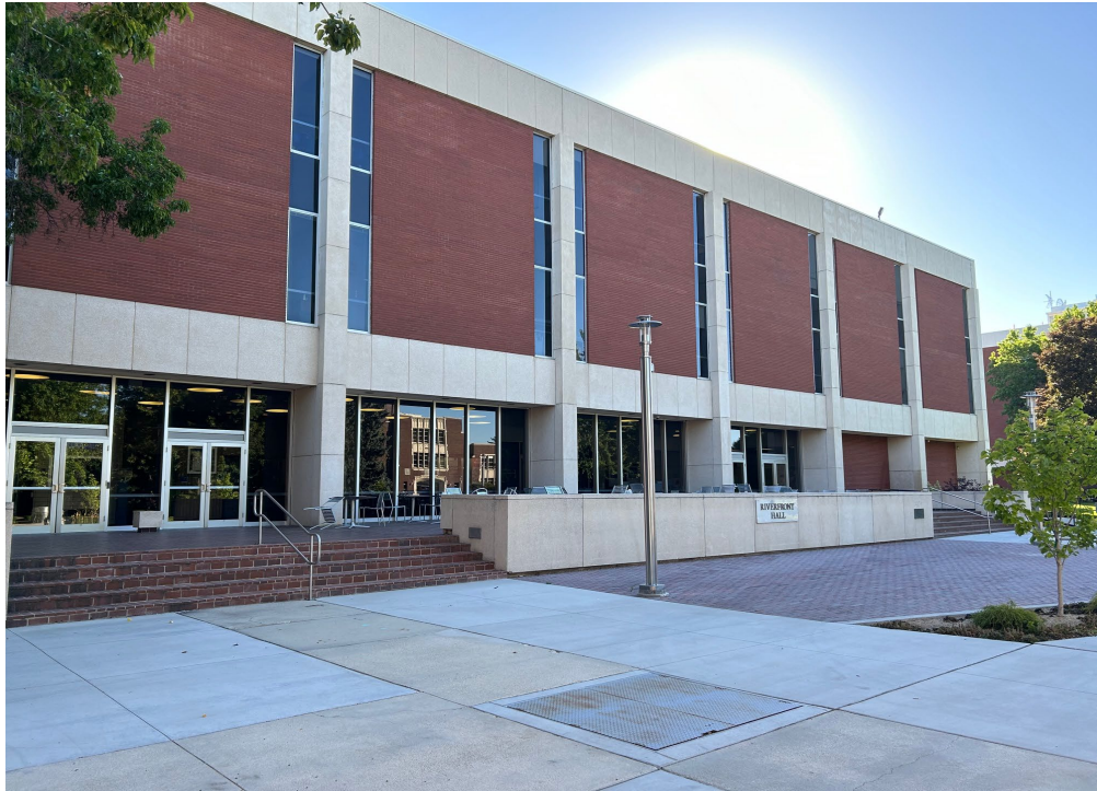
Fig. 1: Riverfront Hall Facade
