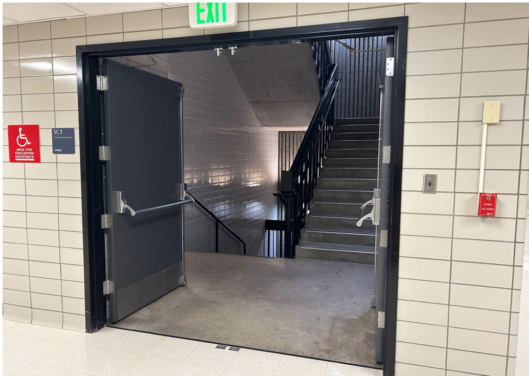
Fig. 4: Poor Lighting in Stairwells
